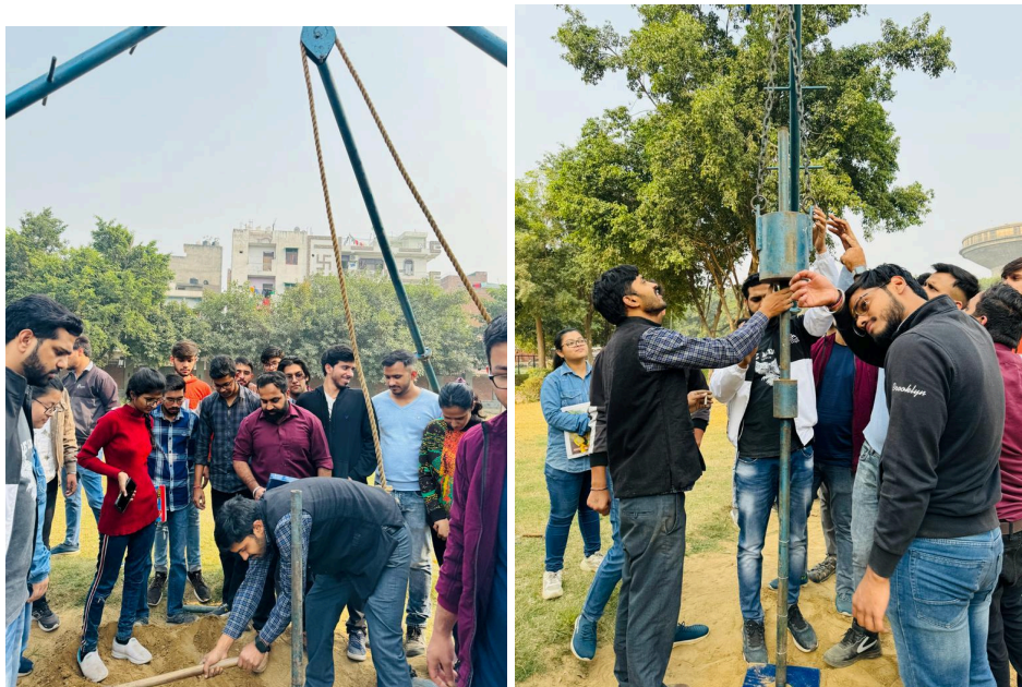
Glimpse of Soil Testing using SPT
