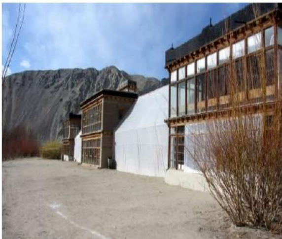
The southern face of the main building of SECMOL Alternative School is all windows as it gets maximum sunrise to sunset exposure in winters.
