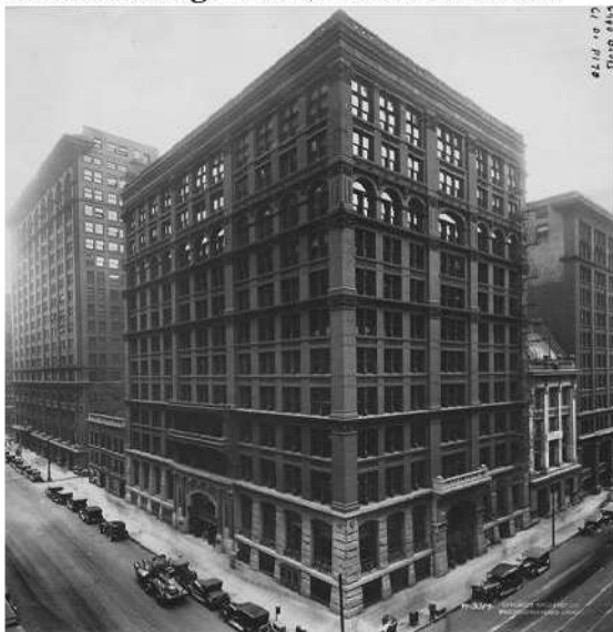
Chicago's Home Insurance Building is widely considered to be the world's first modern skyscraper.
